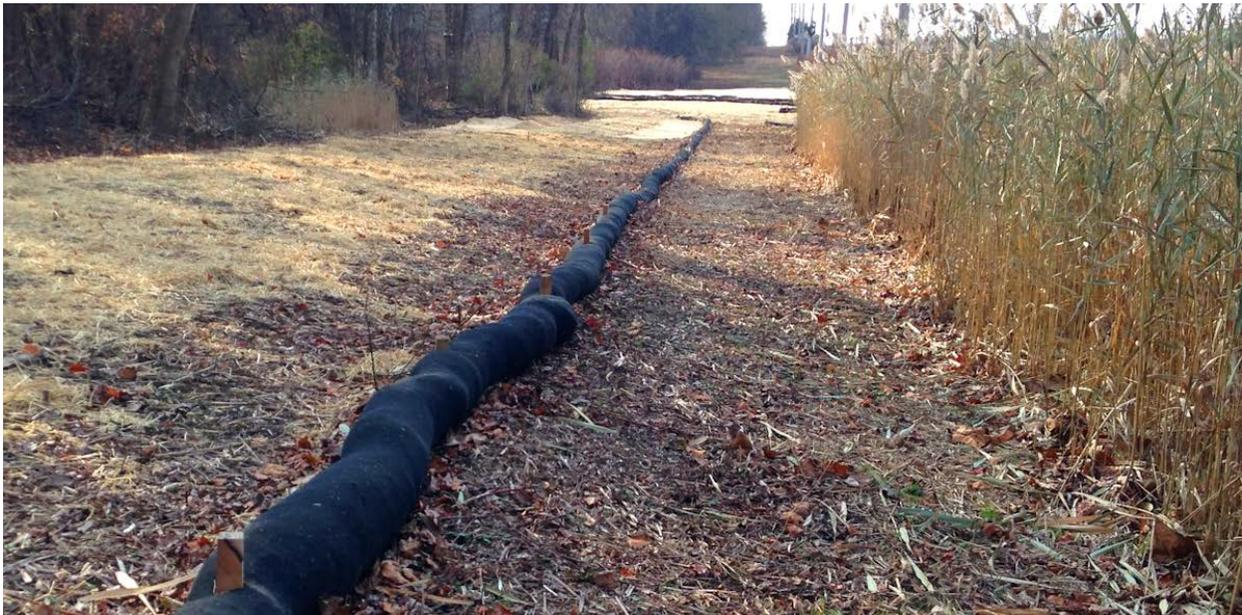
“Silt sock” made from a porous fabric tube filled with mulch filters stormwater running off construction sites to help keep sediment out of streams and wetlands.
