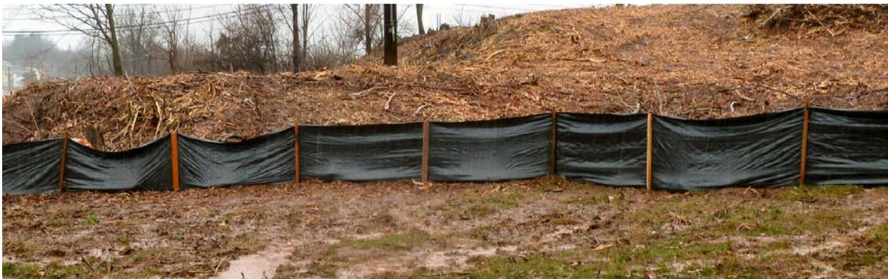
Silt fencing, if properly installed, can reduce sediment runoff from construction sites or other disturbed areas lacking vegetation.
